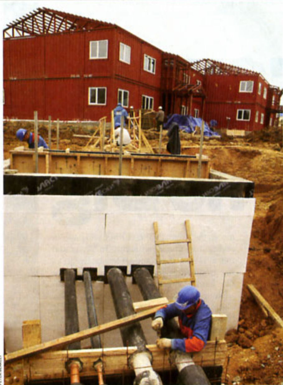
BOOMTOWN: Breaking ground on 100 new employee housing units
